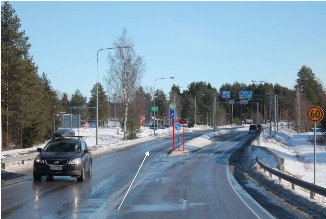
Pos 6/Pic 10. Road 8. Continue straight on counter lane. https://goo.gl/maps/zBqM1gULQySmSoFh6 . Marked sign need to be removed.
