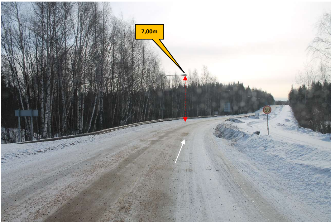
Pos 2/Pic 2. KoksaaMontie. Continue straight. https://goo.gl/maps/cbCiVDtjACptdCDj6 . Marked lamp post height to be rechecked before transports.
