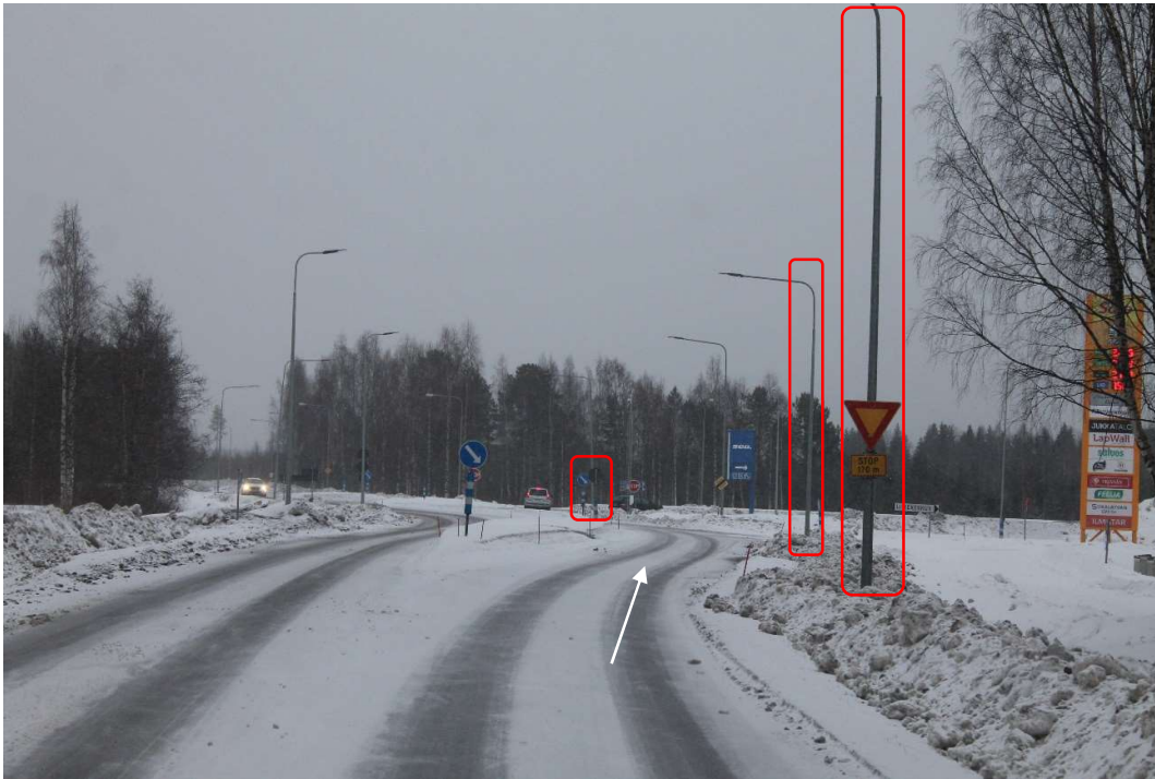
Pos 17/Pic 27. Road 88. https://goo.gl/maps/UnHpVqDEzfYUMwou7 Marked lamp posts and signs need to be removed.
