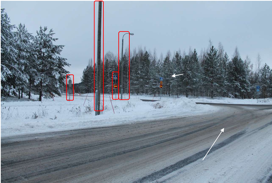
Pos 27/Pic 47. Turning from road 16222 (Tervakankaantie) toward road 5. Need to use counter lane ramp down to road 5. Marked lamp post and sign need to be removed.
