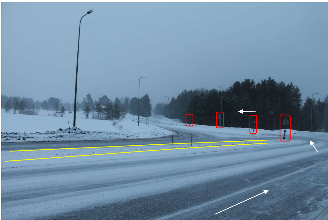
Pos 16/Pic 26. Turning from road 4 toward road 88. Marked signs need to be removed. Marked area need to be filled.
