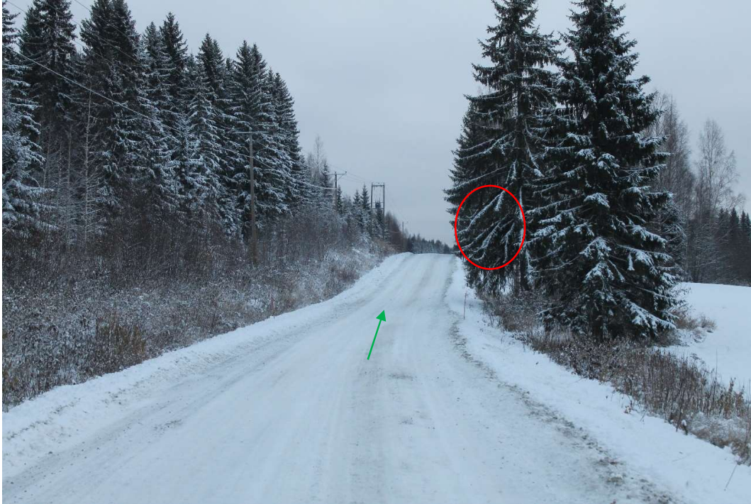
Pos 40/Pic 75. Road 16235 (Keskimmäisentie). https://maps.app.goo.gl/iUVkNZ8KkWbBB0779 Marked tree branches need to cut. Crest, road need to be levelled. Road need to be fixed according to specifications for site roads. Green arrow points driving direction for Entrance B.
