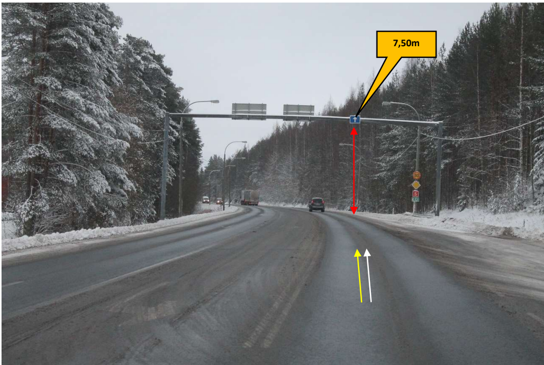
Pos 30/Pic 56. Road 5. https://maps.app.goo.gl/T6fZLTpE7Ej9am6i9 Info : Portal height 7,50m. White arrow points driving direction for route 1. Yellow arrow points driving direction for route 2.
