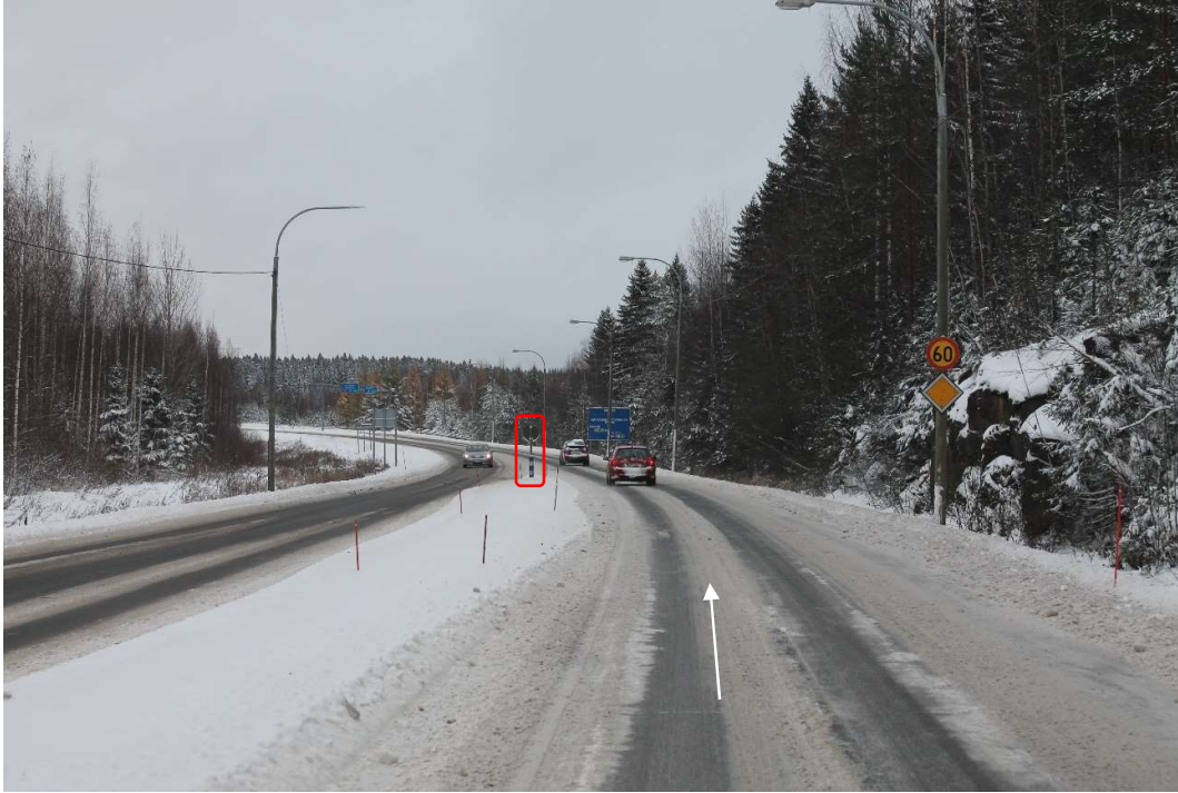
Pos 21/Pic 35. Road 27. https://maps.app.goo.gl/vm4ZiPHRZGkrWaVY9 Marked sign need to be removed.
