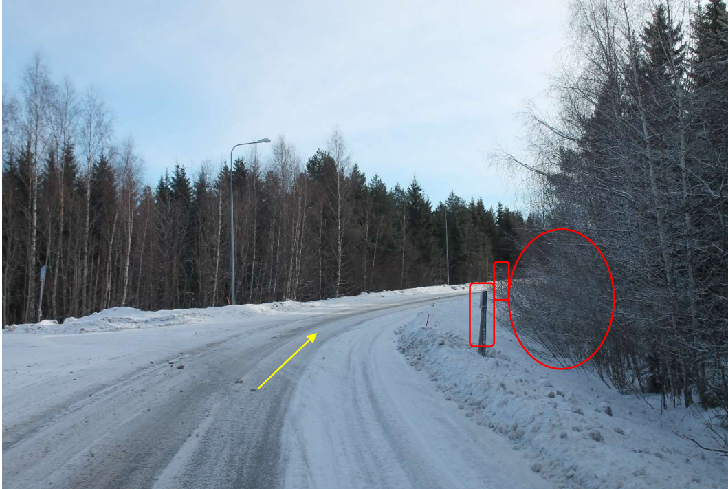
Pos 44/Pic 85. Lapaluodontie. Marked signs to be removed. Marked bush/trees need to cut.
