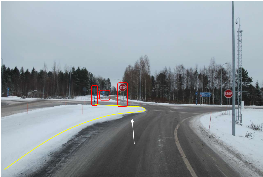
Pos 17/Pic 29. Road 88. Marked signs need to be removed. Marked area need to be filled and drivable.
