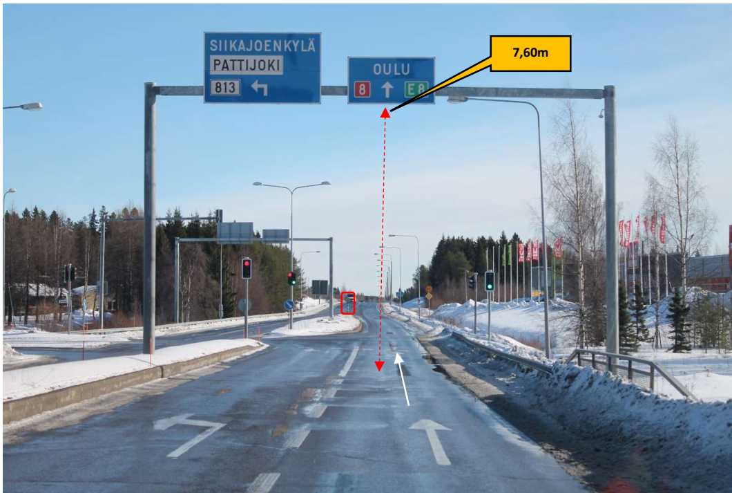
Pos 7/Pic 12. Road 8. https://goo.gl/maps/pPpDXCU26rpkJyuu5 . Marked sign need to be removed.
