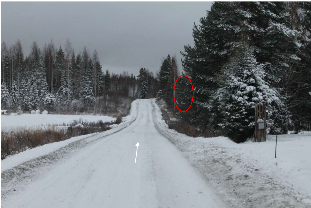
Pos 33/Pic 62. Road 16235 (Keskimmäisentie). https://maps.app.goo.gl/TpruVuuPDgdp6VWZA Road need to be levelled. Marked tree branches need to cut. Road need to be fixed according to specifications for site roads.
