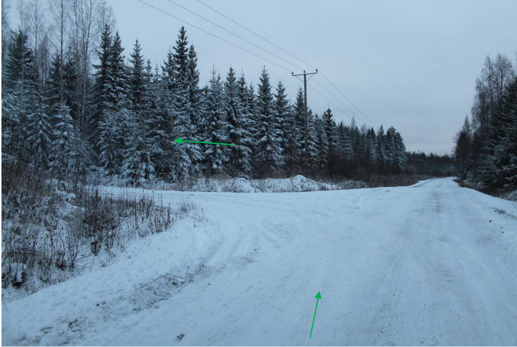
Pos 42/Pic 81. Turning from road 16235 (Keskimmäisentie) toward site area. Crest, road need to be levelled. Road need to be fixed according to specifications for site roads. Site entrance to be build according to specifications for site roads. Green arrow points driving direction for Entrance B.
