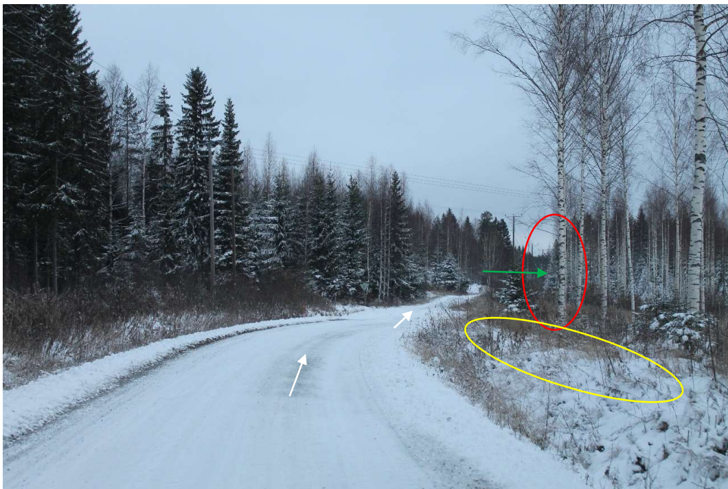
Pos 38/Pic 70. Turning from road 16235 (Keskimmäisentie) toward site area. https://maps.app.goo.gl/SwhhPjhhk6GjWmU89 This is plan A for site entrance. Marked trees need to cut. Oversail area need to be free in inner curve. Site entrance to be build according to specifications for site roads. Green arrow points driving direction for Entrance B.
