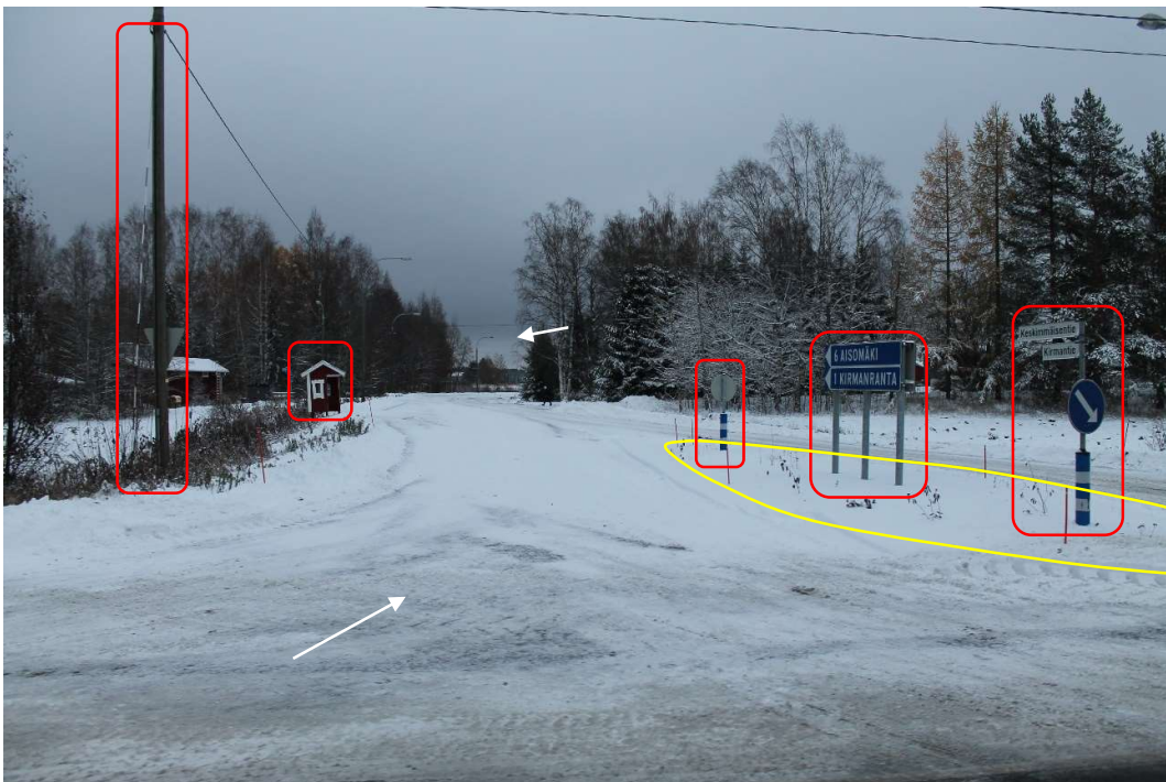
Pos 31/Pic 60. Turning from road 5 toward road 16235 (Keskimmäisentie). Marked signs, bus shelter and lamp post need to be removed. Marked traffic island need to be flat and drivable.
