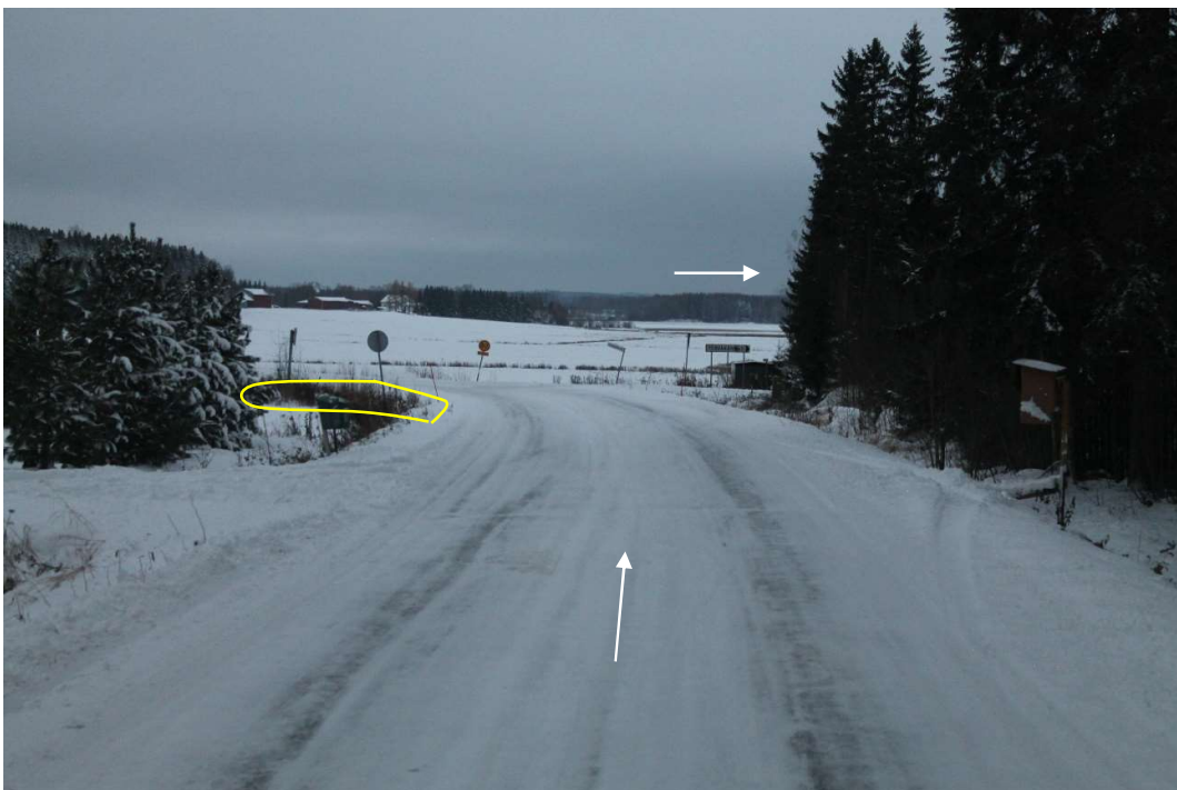
Pos 25/Pic 42. Turning from road 16229 (Koukkujoentie) toward road 16222 (Tervakankaantie). https://maps.app.goo.gl/vT9h5FcDtytrXpPW6 Markes area need to be filled and drivable. Privat land in inner curve.
