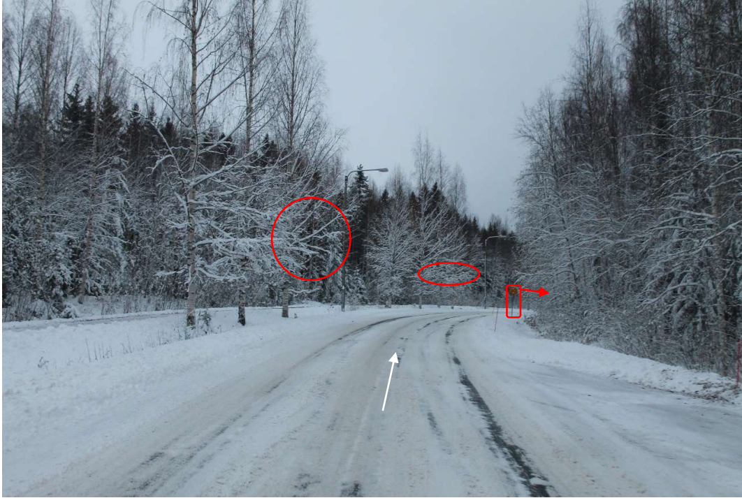
Pos 26/Pic 45. Road 16222 (Tervakankaantie). https://maps.app.goo.gl/gRJBRCQuPe153AN8 Marked tree branches need to cut. Marked sign need to be removed.
