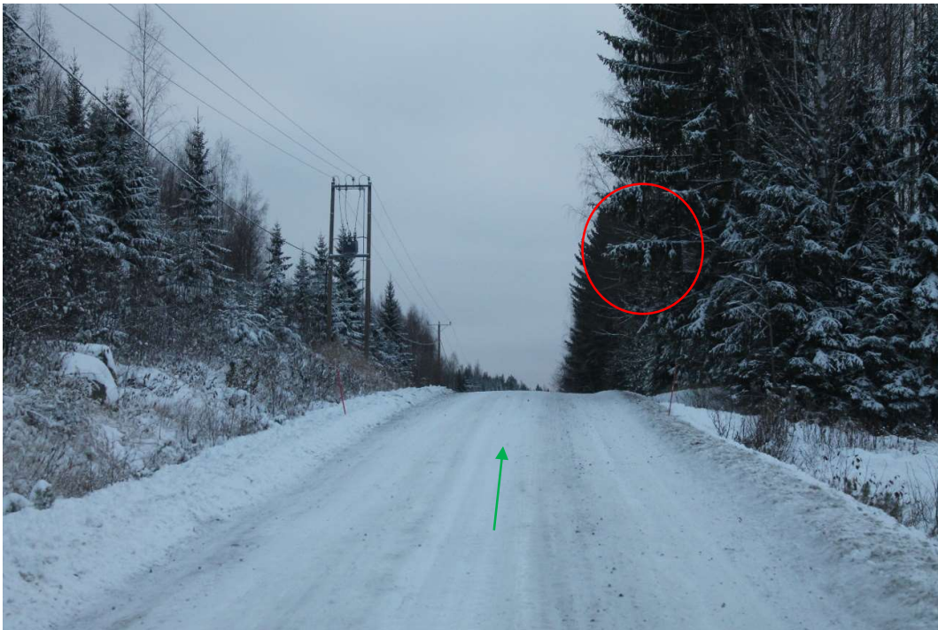
Pos 40/Pic 76. Road 16235 (Keskimmäisentie). Marked tree branches need to cut. Crest, road need to be levelled. Road need to be fixed according to specifications for site roads. Green arrow points driving direction for Entrance B.
