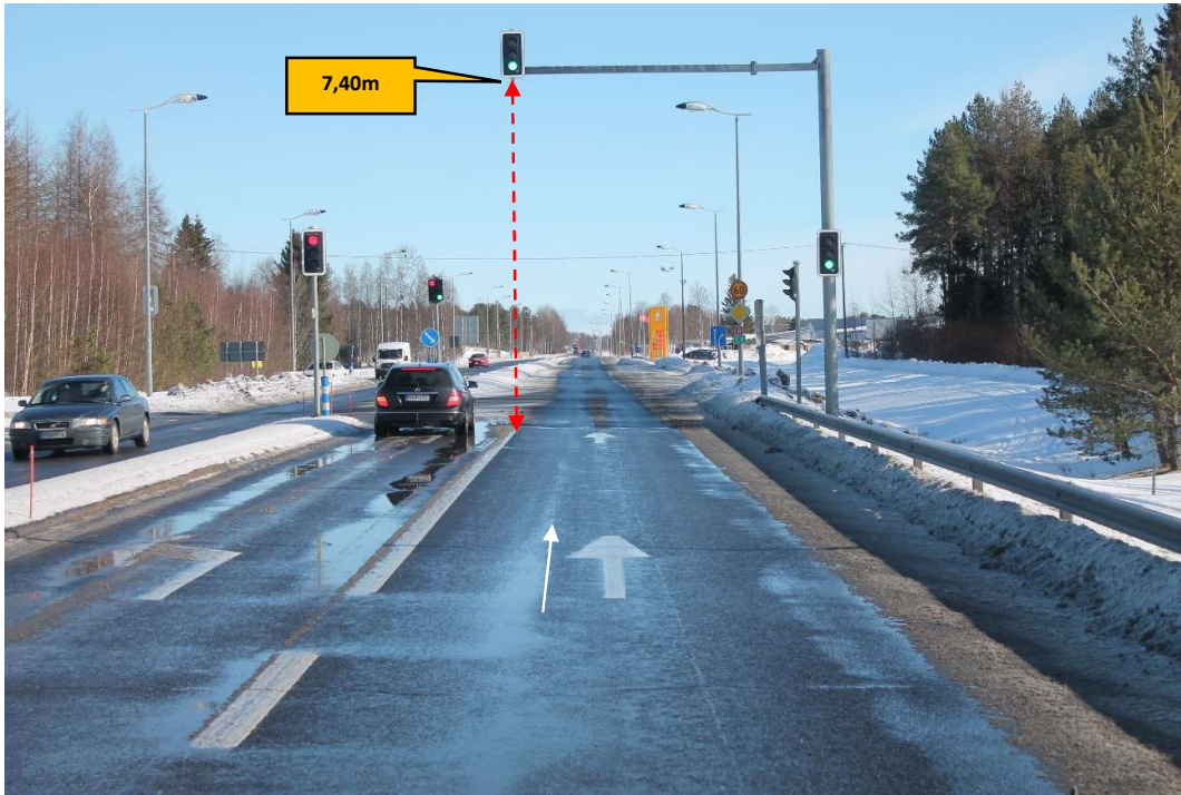
Pos 12/Pic 19. Road 8. https://goo.gl/maps/Mg36qefhwnvMgzZ57
