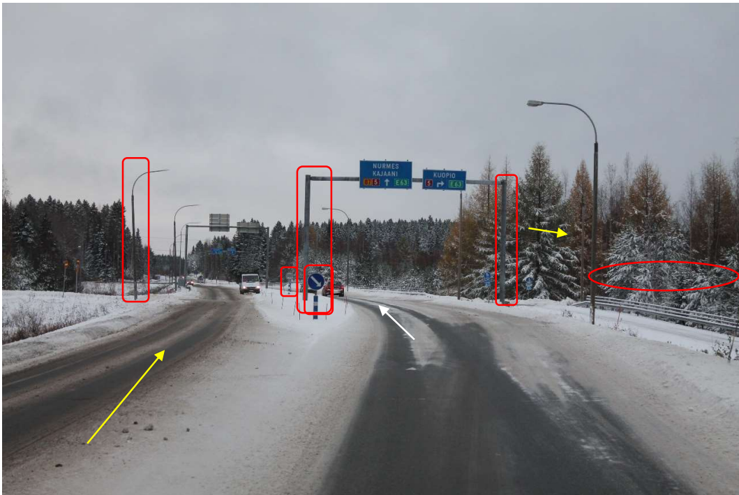
Pos 22/Pic 36. Road 27/ road 87. https://maps.app.goo.gl/z7jdHKeBPhhYG2E58 Blades turning from road 27 toward road 5. Yellow arrow points driving direction for route 2 Oversail area need to be flat and free on right side. Marked signs and pole need to be removed. White arrow points driving direction for route 1.
