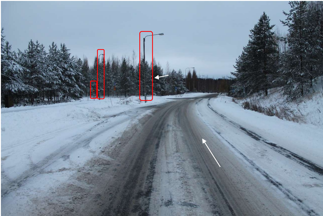
Pos 27/Pic 46. Turning from road 16222 (Tervakankaantie) toward road 5. https://maps.app.goo.gl/qX2bfEkjKnxyS7i56 Need to use counter lane ramp down to road 5. Marked lamp post and sign need to be removed.
