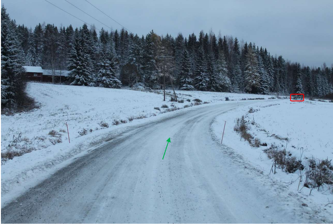
Pos 39/Pic 73. Road 16235 (Keskimmäisentie). https://maps.app.goo.gl/6cFueGLmQTr5ZbLE9 Road need to be levelled. Road need to be fixed according to specifications for site roads. Marked mail box need to be removed. Green arrow points driving direction for Entrance B.
