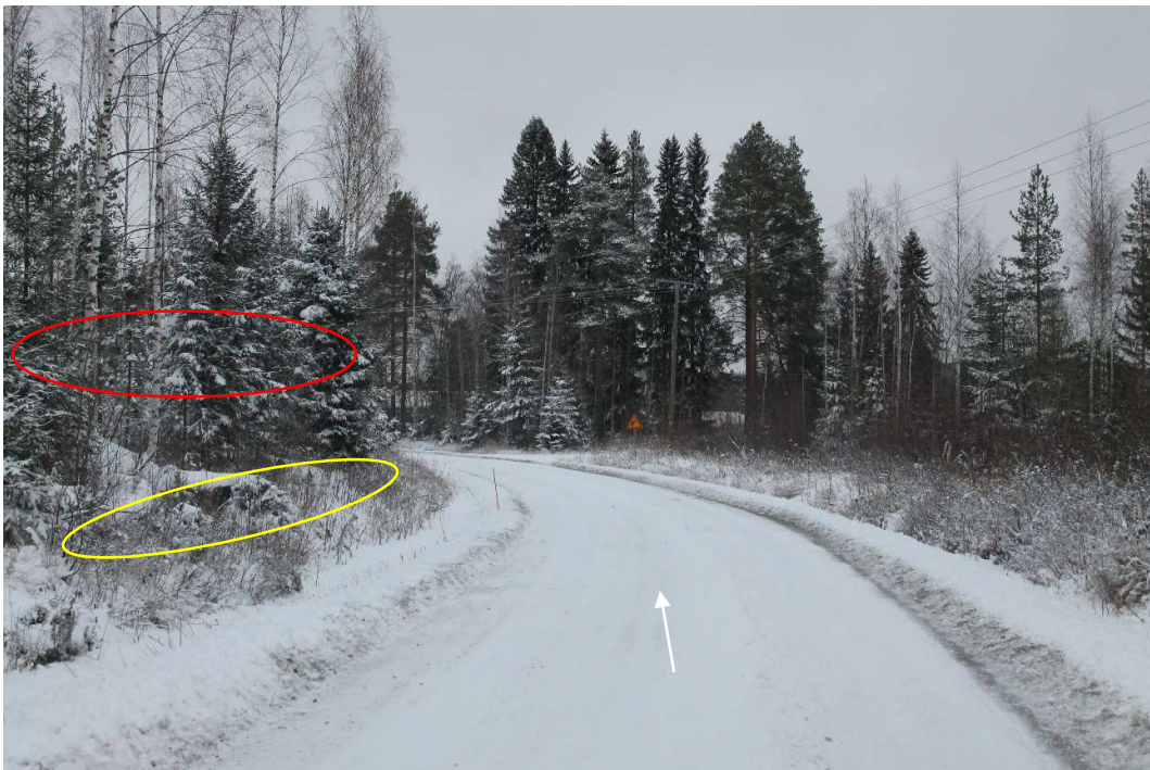
Pos 36/Pic 68. Road 16235 (Keskimmäisentie). https://maps.app.goo.gl/5d8XuhNKt1G3e9q68 Marked trees need to cut. Oversail area need to be free in inner curve. Road need to be levelled. Road need to be fixed according to specifications for site roads.
