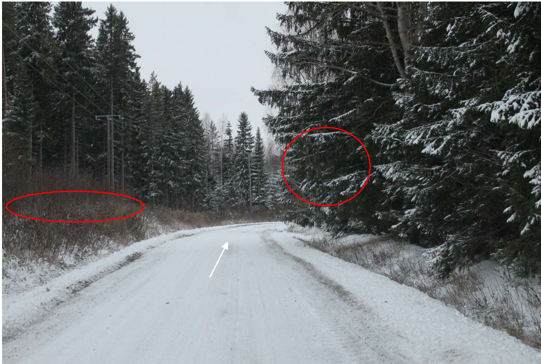
Pos 37/Pic 69. Road 16235 (Keskimmäisentie). https://maps.app.goo.gl/abNpDz9job1UJYQ69 Marked trees need to cut. Oversail area need to be free in inner curve. Road need to be levelled. Road need to be fixed according to specifications for site roads.
