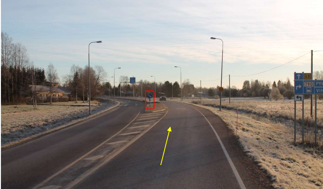
Pos 47/Pic 91. Road 88. https://goo.gl/maps/9j58sMbdbnfWDuyP9 Marked sign need to be removed.
