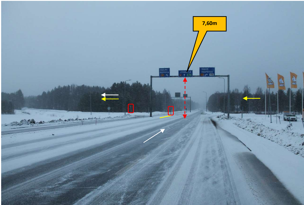
Pos 16/Pic 25. Turning from road 4 toward road 88. https://goo.gl/maps/qqsMmTAftgPnDaHi7 Marked signs need to be removed. Marked area need to be filled. Yellow arrow points driving direction for route 2.
