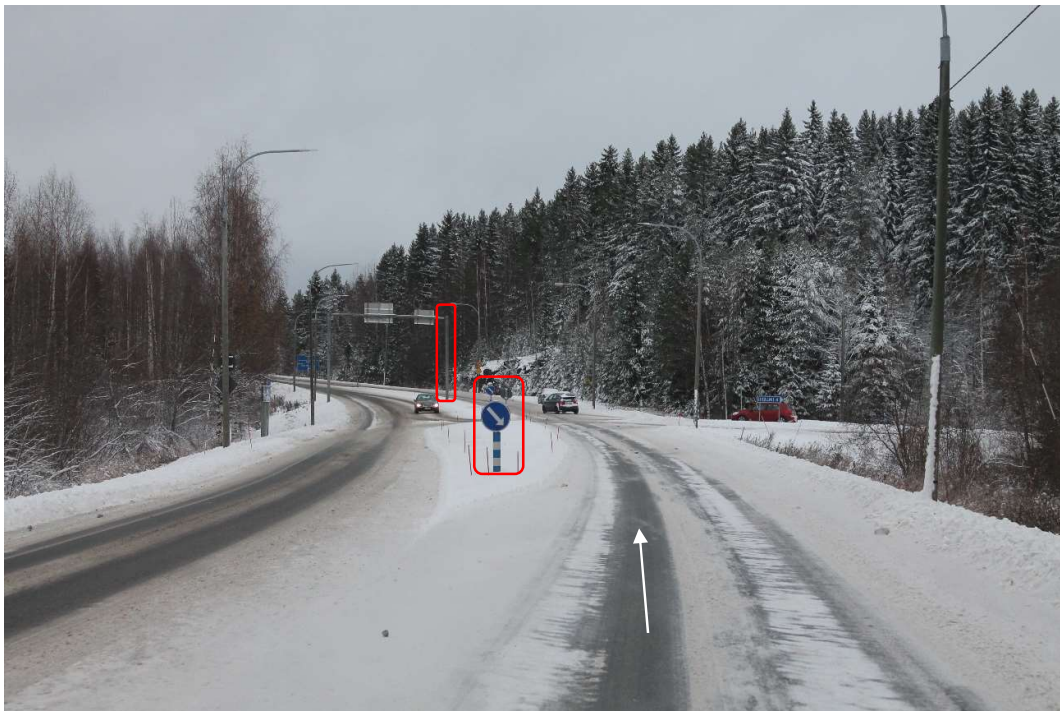
Pos 21/Pic 34. Road 27. https://maps.app.goo.gl/vm4ZiPHRZGkrWaVY9 Marked signs and portal pole need to be removed.
