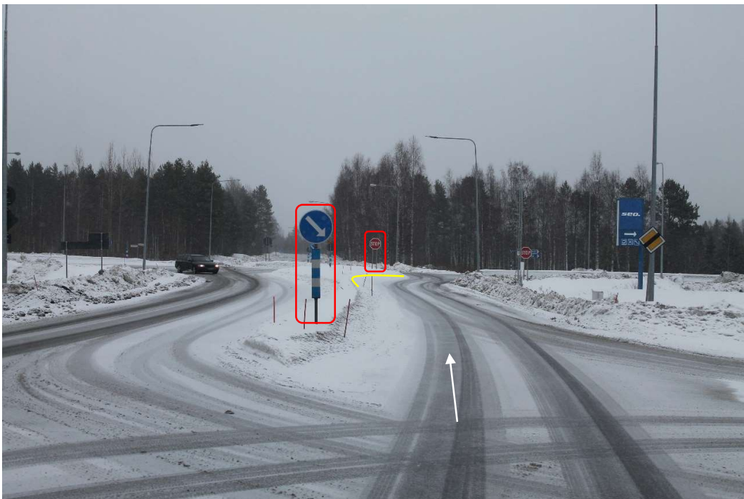
Pos 17/Pic 28. Road 88. Marked signs need to be removed. Marked area need to be filled and drivable.
