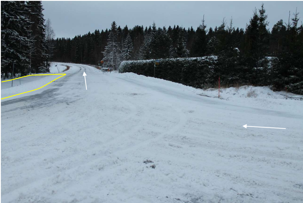
Pos 25/Pic 44. Turning from road 16229 (Koukkujoentie) toward road 16222 (Tervakankaantie). Marked area need to be filled and drivable.
