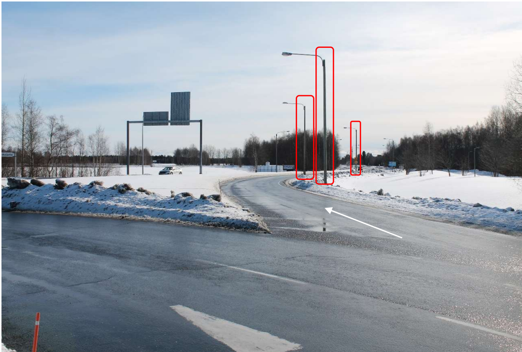
Pos 14/Pic 23. Turning from road 8 toward road 4. Marked lamp posts need to be removed.
