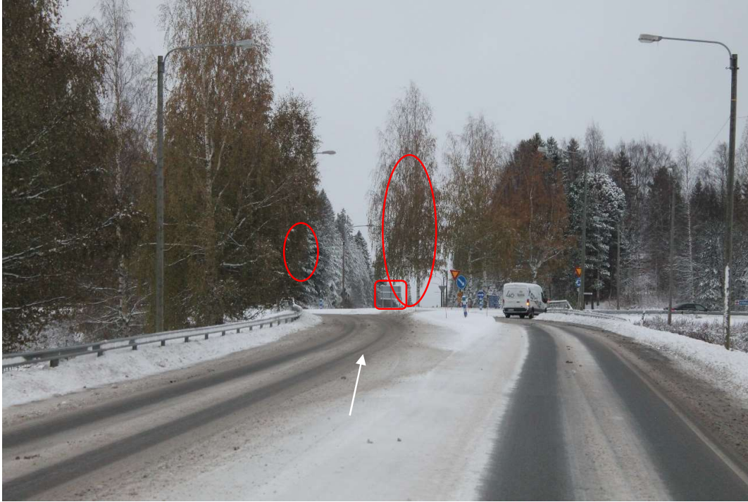
Pos 19/Pic 31. Roundabout road 27. https://maps.app.goo.gl/BE7ZVfhP9CcpUvRd9 Marked sign need to be removed. Marked trees and tree branches above of the road need to cut.
