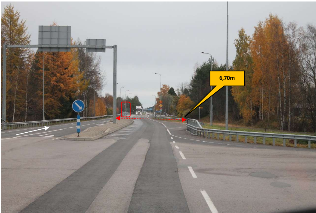
Pos 8/Pic 14. Road 8. https://goo.gl/maps/fLBjdYMtXjLyqj1Z9 . Need to use counter lane. Marked sign need to be removed.
